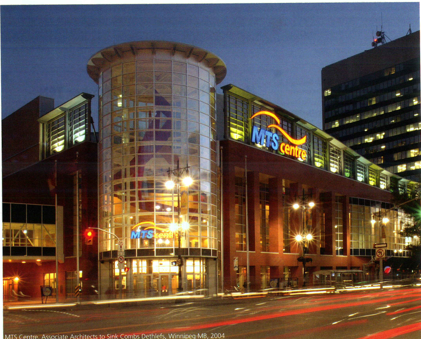
MTS Centre, Associate Architects to Sink Combs Dethlefs, Winnipeg MB, 2004
